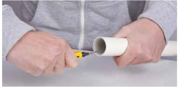
Fig. 7: Make a visible edge all over the pipe end (inside the pipe) by using a universal beveling tool.
