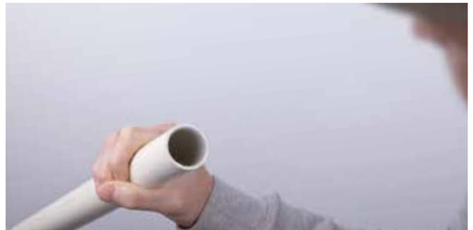
Fig. 9 Make an optical check of pipe end if the chamfer is running around the pipe and if the parts are free from impurities.
