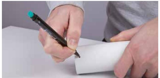
Fig. 11: Mark the welding insertion depth on the pipe end.
